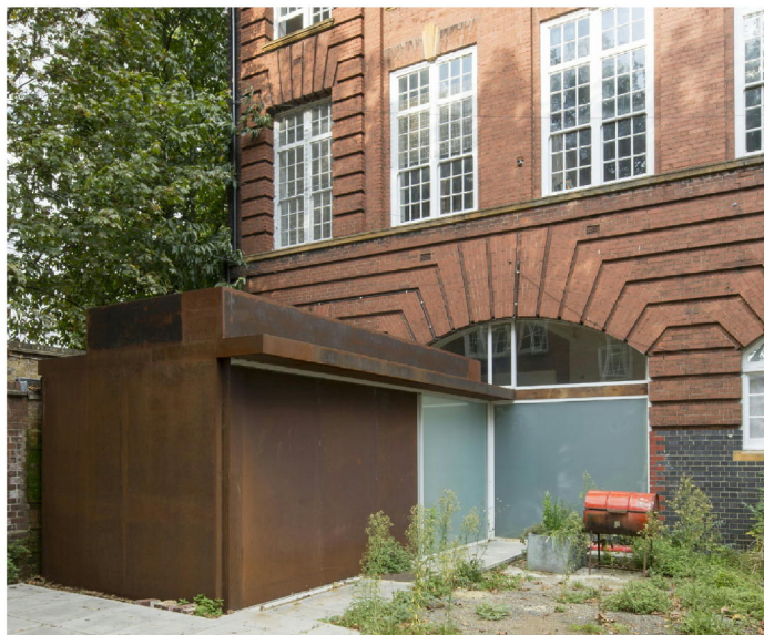
Left: Studio 3, a COR-TEN extension to the Grade II Listed Stepney Jewish Primary & Infants School London E1, designed by Friend and Company Architects (2014).
