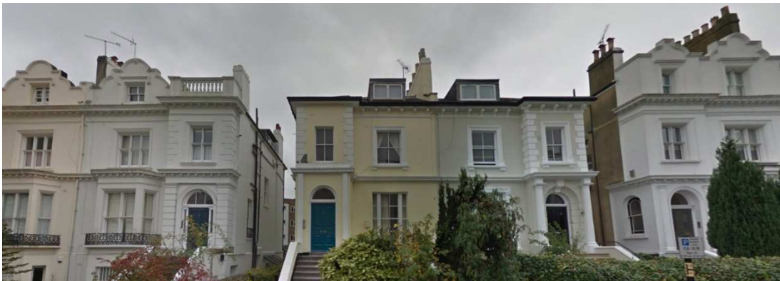
Typical architectural character of the conservation area
