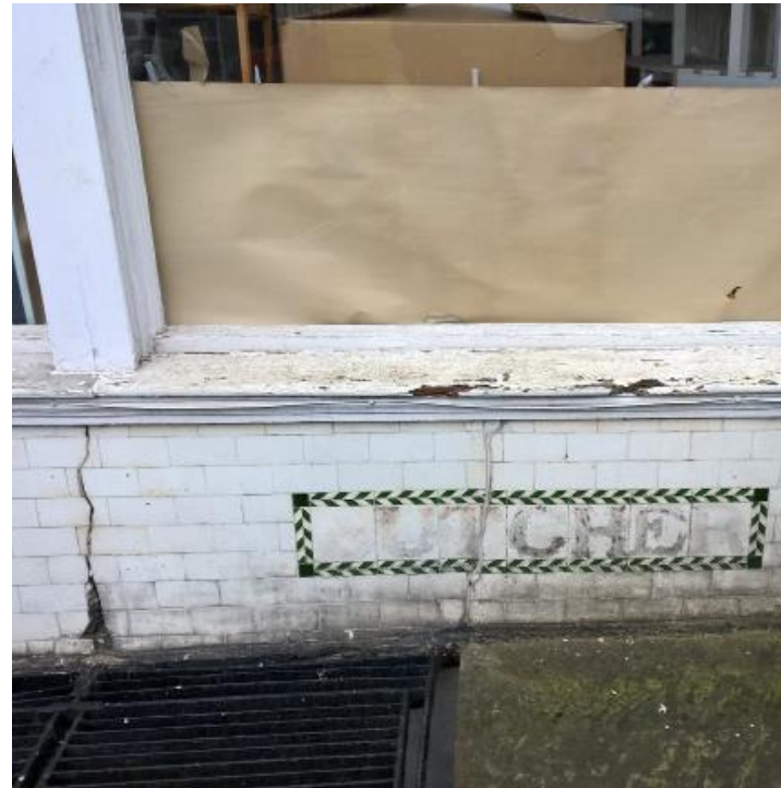
Original tiling / signage to shopfront
