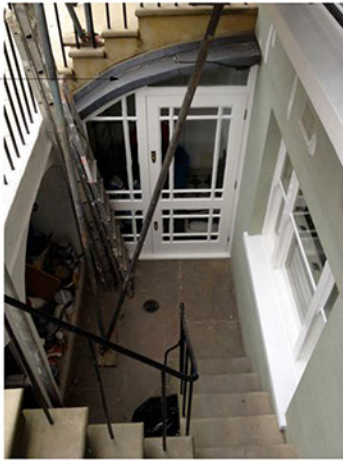
PHOTO OF LIGHTWELL AT NO. 23 FITZROY ROAD
