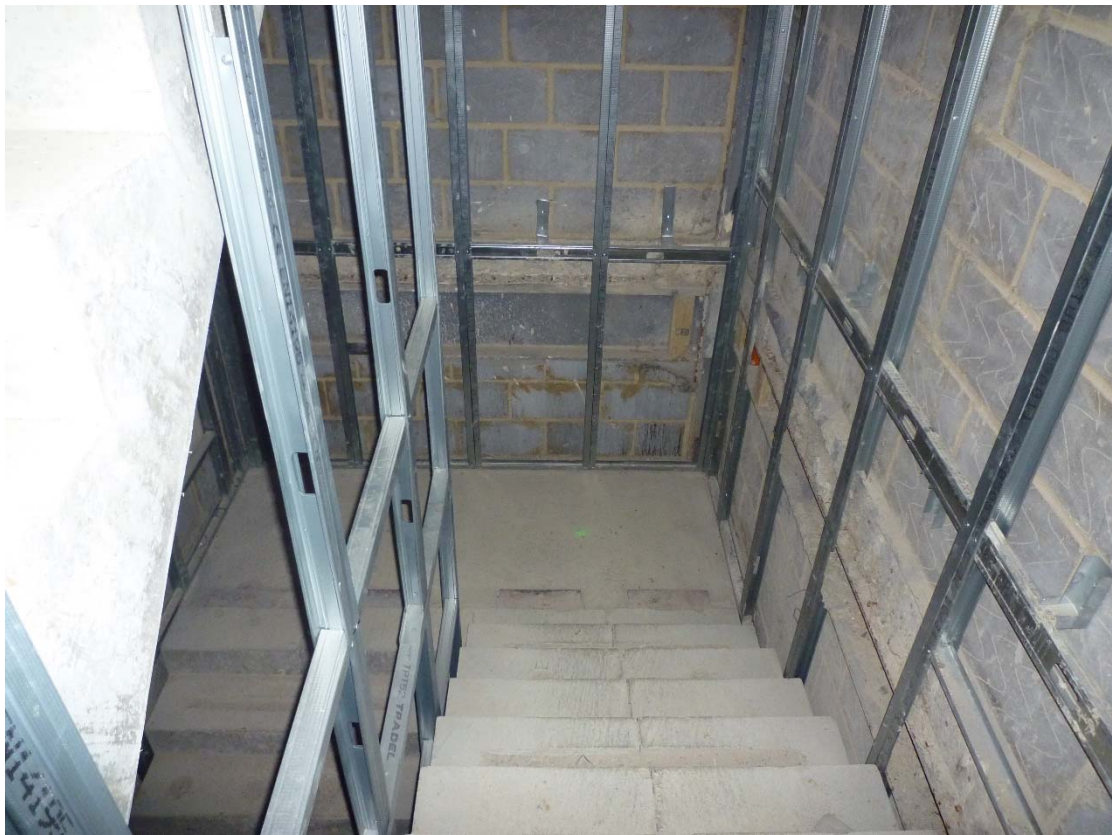
Fig.6 the new stair from ground floor to basement
