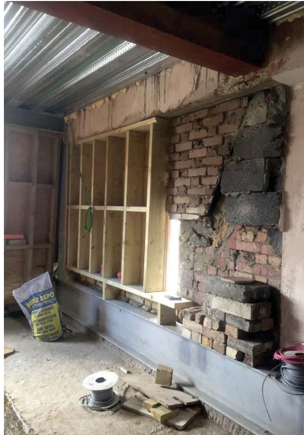
05 New steel structure as per 2015/3149/P consent
