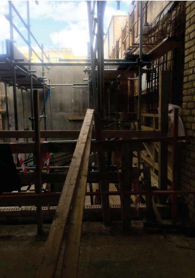
01 Rear Elevation has been demolished and reinstated as per 2015/3149/P consent
