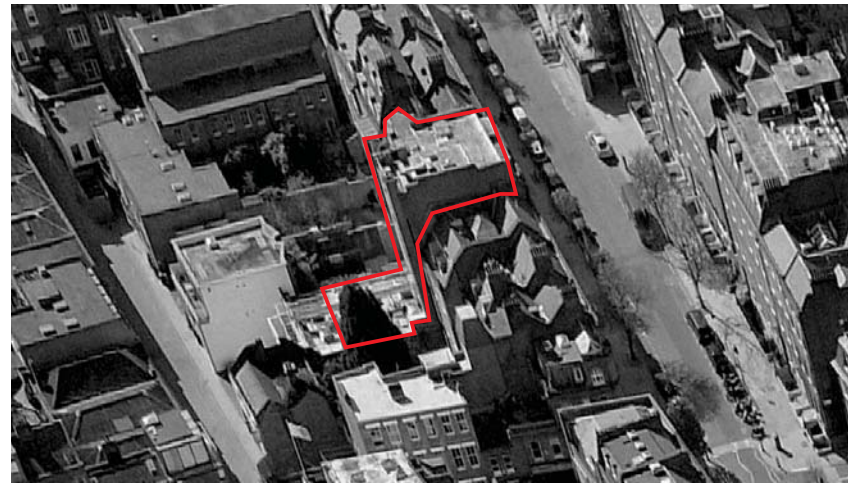
04 Aerial View looking South
