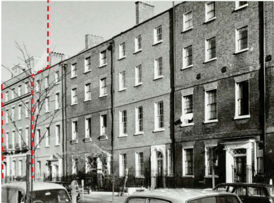
1965 Historic Photograph 6-9 John Street Rear Elevation
