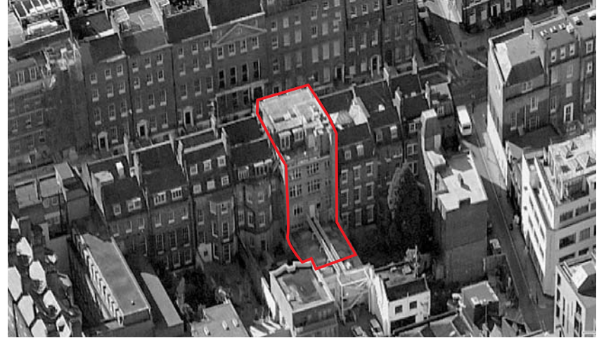
02 Aerial View looking West
