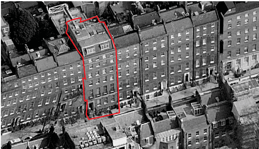
03 Aerial View looking East
