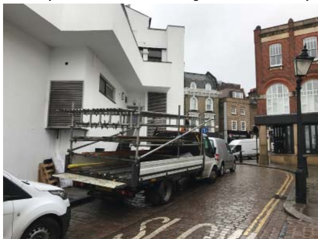
Scaffolding delivery along Back Lane
