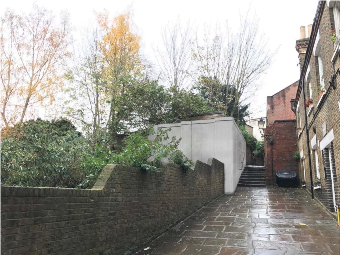
Indicative visualisation of what hoarding could be on Streatley Place Full design to be submitted later by scaffolding contractor for consideration and approval for scaffolding licence from Camden Council
