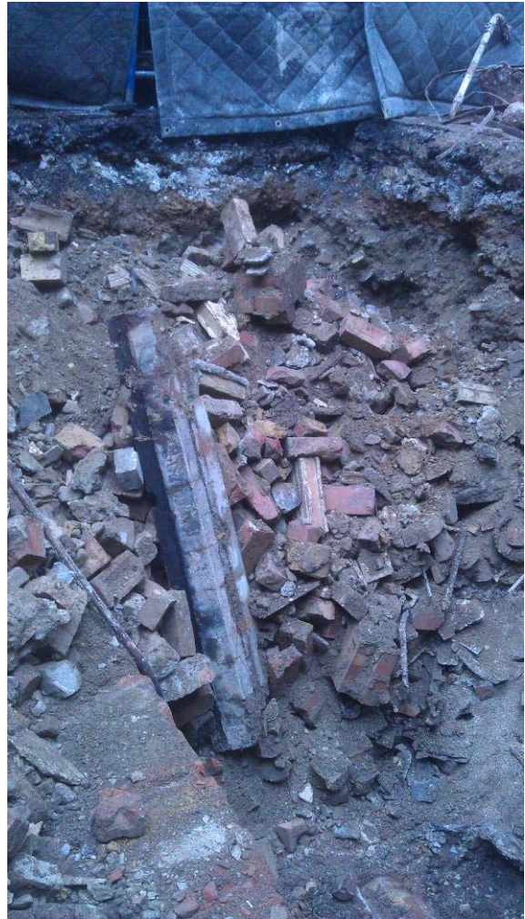
Photo 4 excavation of Southwood yard
