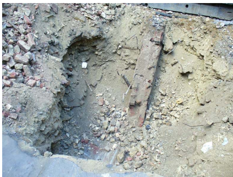
Photo 5 excavation of Southwood yard
