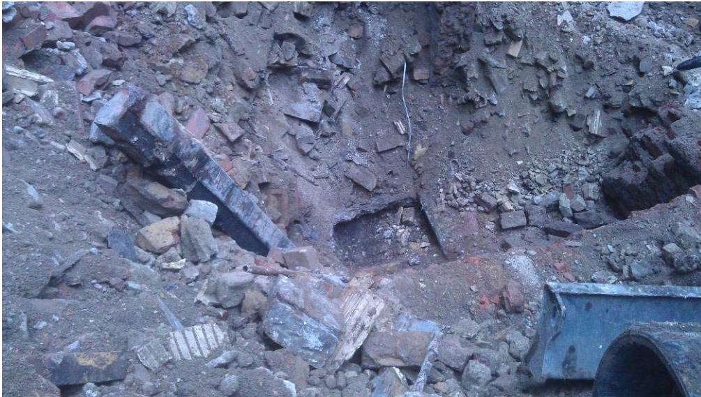
Photo 1 excavation of Southwood Yard
