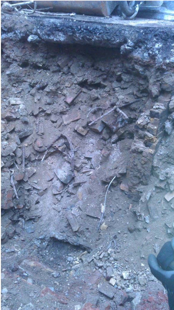
Photo 3 excavation of Southwood Yard
