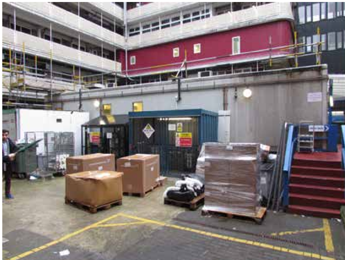
Plate 1: View of the Site Looking East
