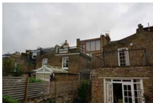
View of existing rear elevation and side passageway
