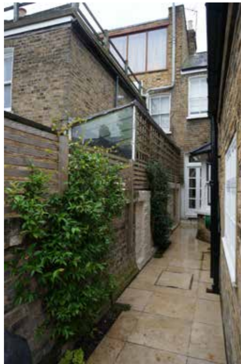
Existing side passageway
