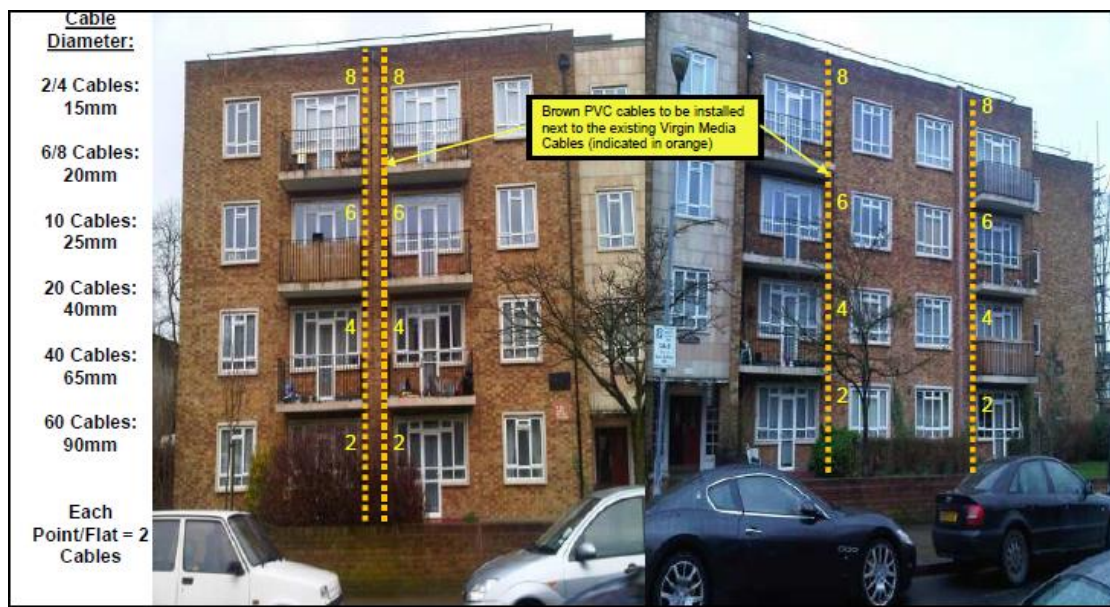
Figures 8 and 9 Extracts from the permitted, submitted drawings for satellite dishes, antenna and external cable runs at Troyes House
