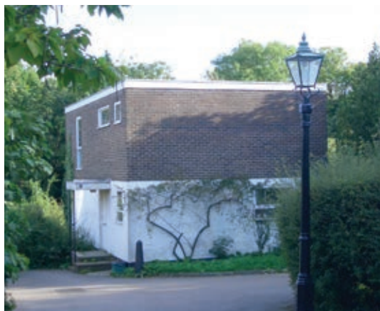
The original house built in 1957.
