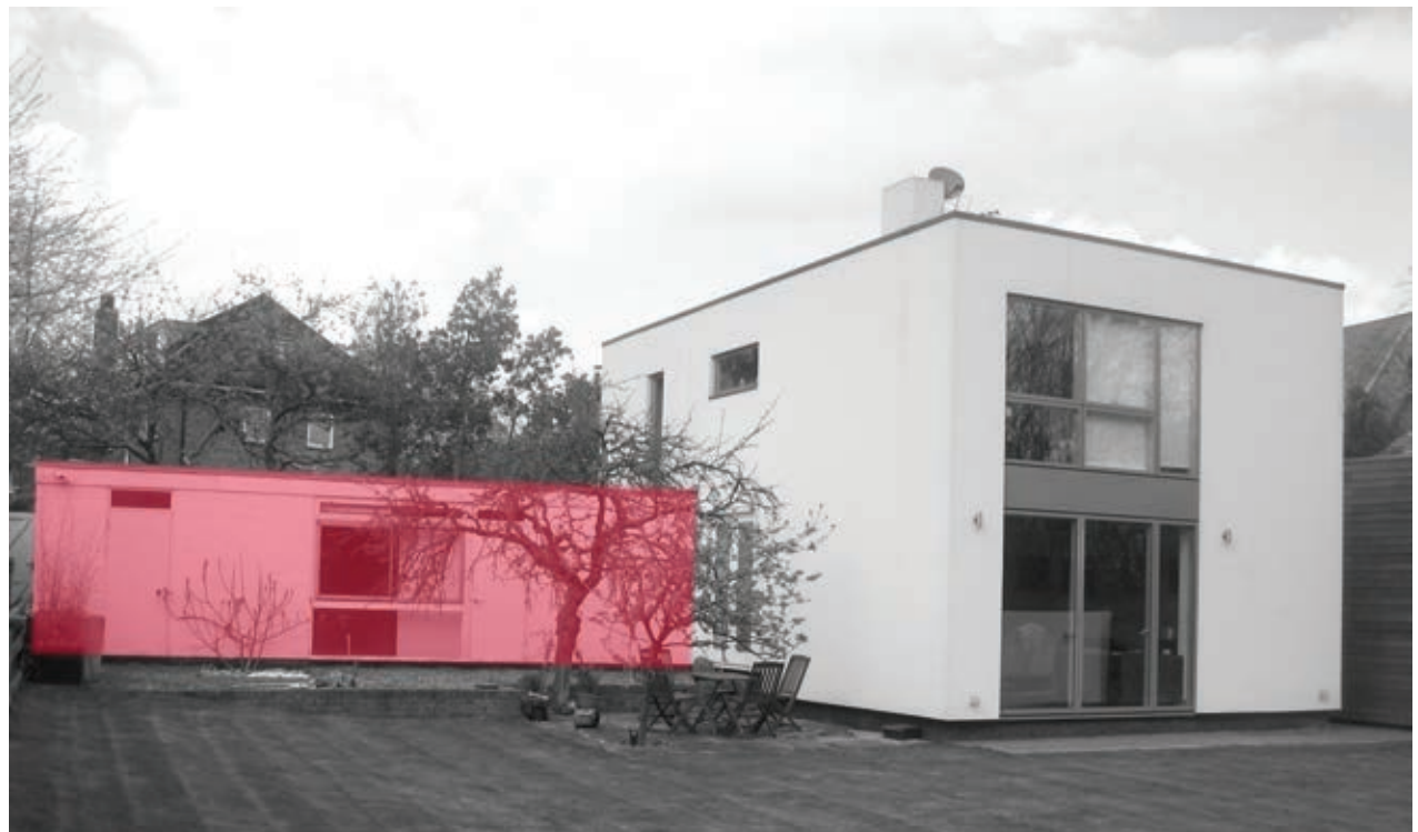
Existing view from garden - wing to be demolished highlighted in red
