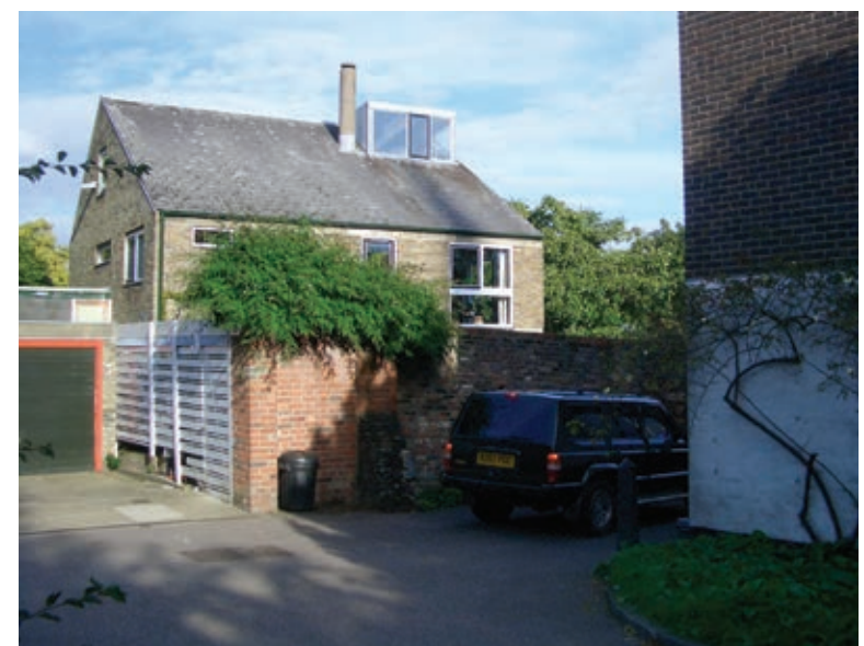
6 Bacon's Lane (designed by Leonard Manasseh), adjoining No 5
