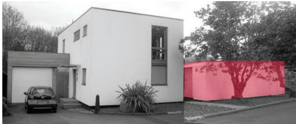
Existing house and wing (highlighted in red) facing onto Bacon's Lane
