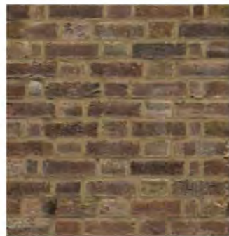
Brickwork to match Existing
