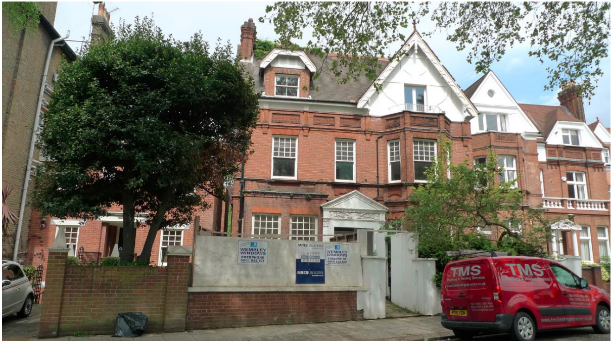
Photo 1: Front elevation of no. 45 Lancaster Grove
