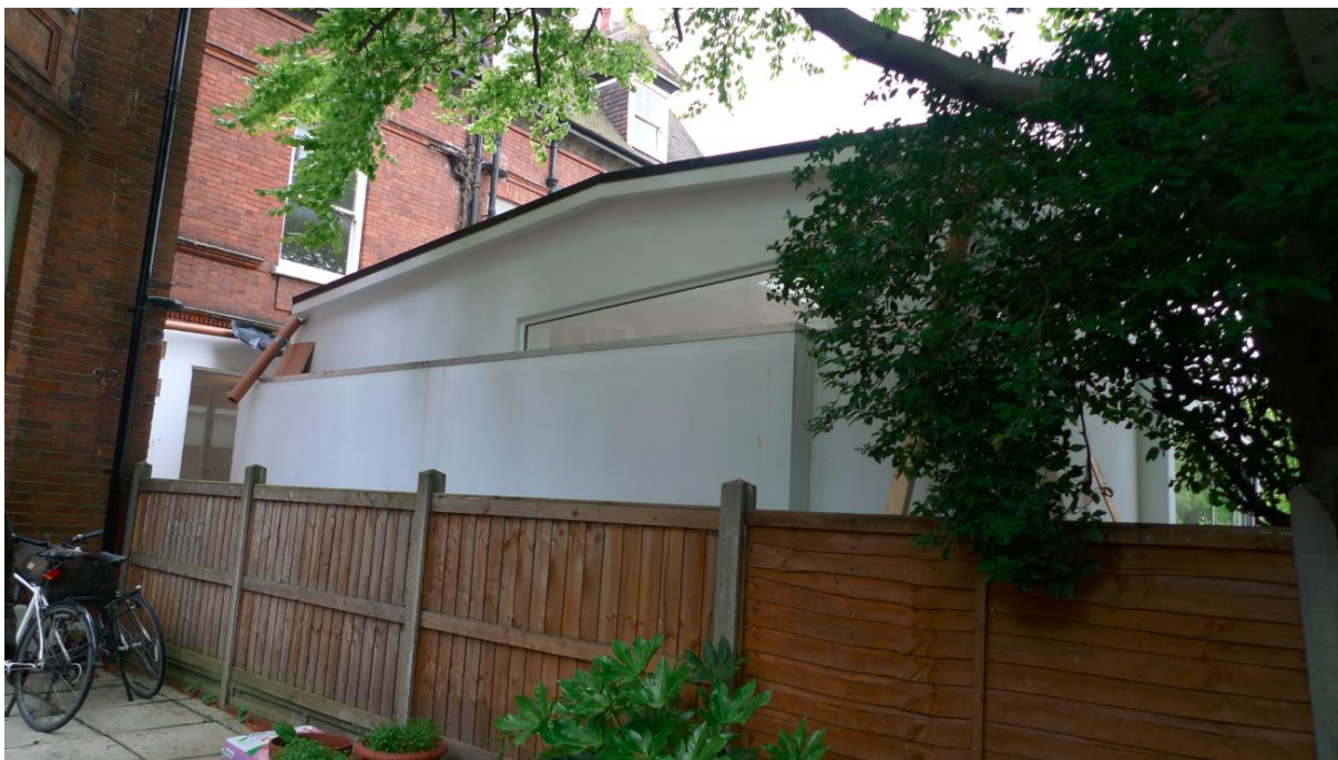
Photo 13: View of eastern side elevation of unauthorised single storey rear extension as part of 2012 scheme that was refused planning permission from neighbouring property at no. 47 Lancaster Grove
