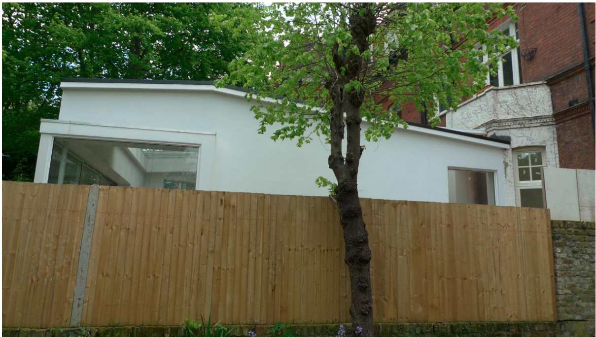
Photo 9: View of western side elevation of existing unauthorised single storey rear extension as part of 2012 scheme that was refused planning permission from garden of no. 43a Lancaster Grove
