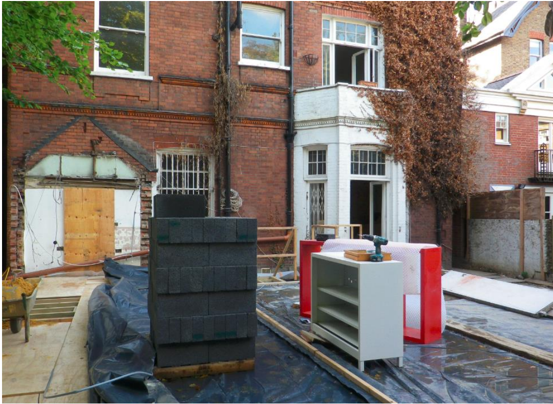
Photo 4: Rear elevation of the property showing the original bay window
