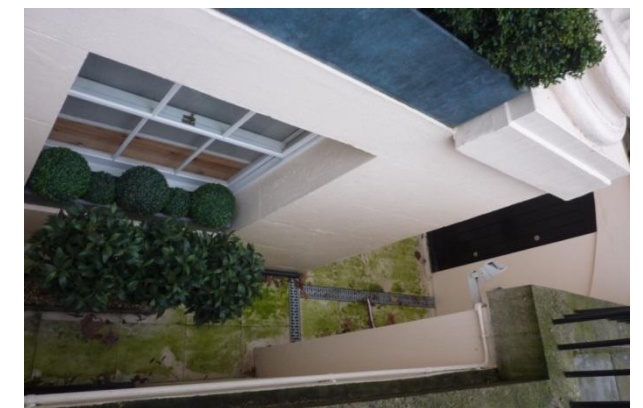
Figure 19: View of No. 36 front light well over railings
