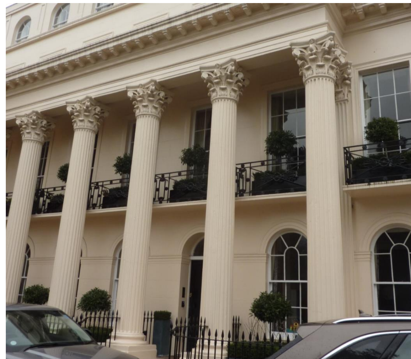
Figure 27: Visibility of proposed opening is obscured by colonnade and deep window reveal
