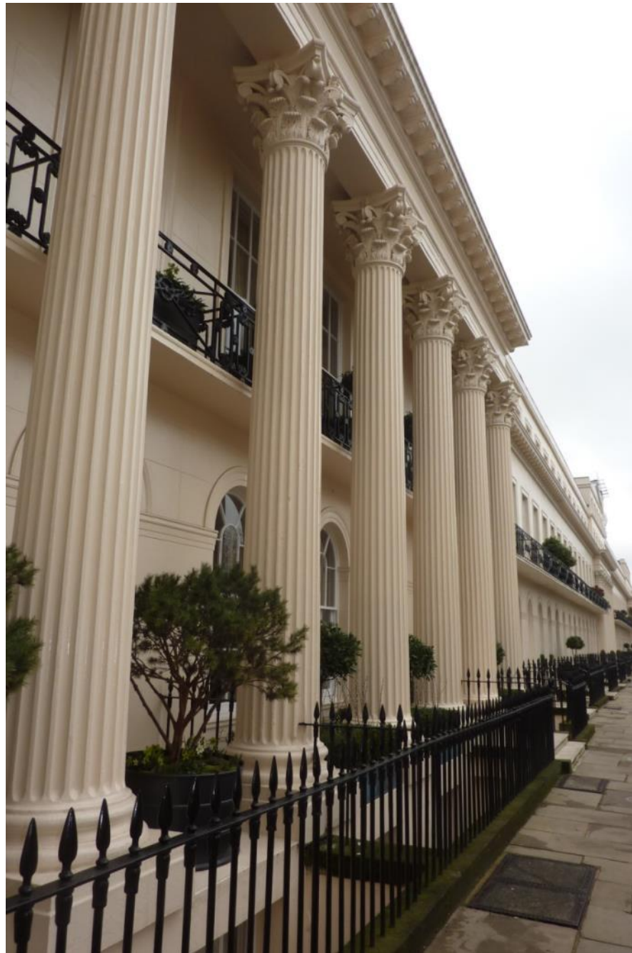
Figure 20: Narrow front light wells to Nos. 36 & 37 preclude a direct view to the light well level and the lower ground floor windows.
