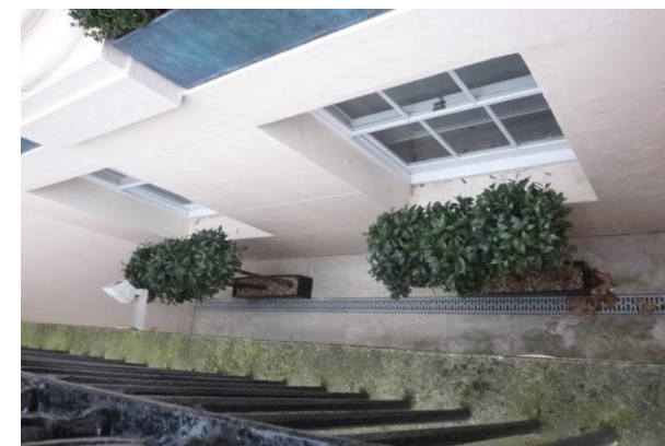
Figure 18: View of No. 37 front light well over railings
