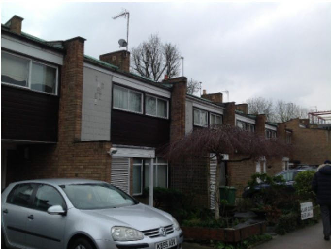
(5) Front elevation #2 (nos. 10 & 11)
