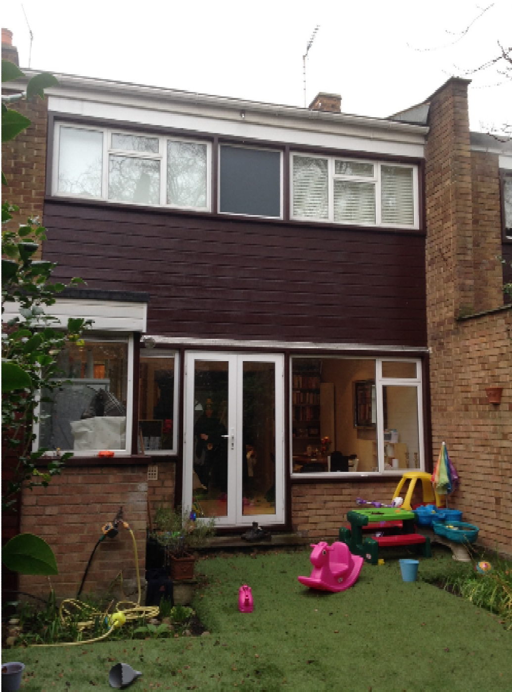
(7) Rear elevation #2 (nos.10&11)
