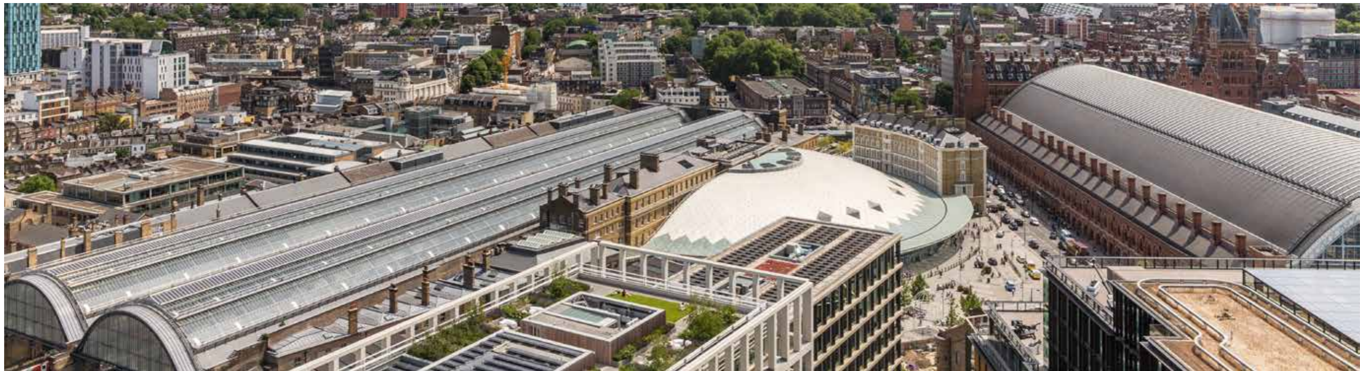
Figure 93: View south towards the city, illustrating the significant linear and repetitive form of the two Grade I listed stations
