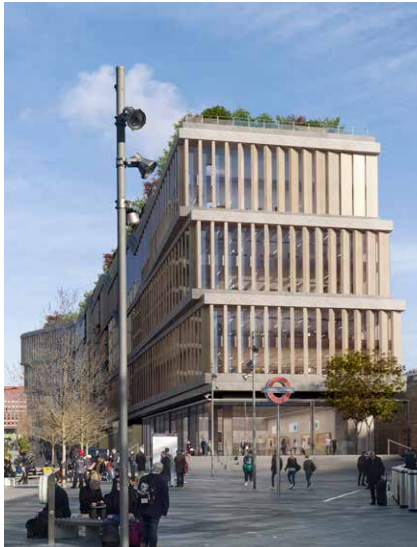
Figure 65: Verified view of the south facade looking north across Battle Bridge Place
