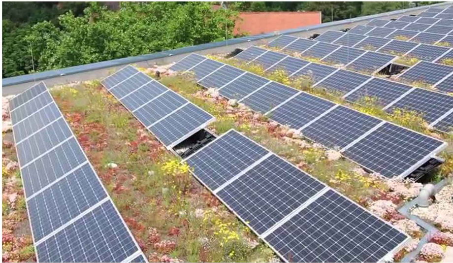
PV Panels on Intensive Green Roof
