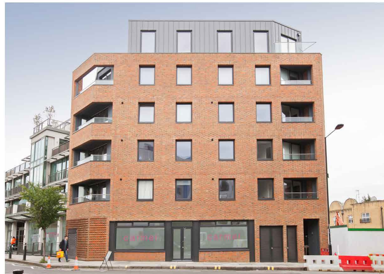
4. 59 Holmes Road; 6 storey, set-back on top storey. [PLANNING REFERENCE : 2012/4056/P] - Erection of a five storey plus basement building comprising light industrial at basement and ground floor levels and residential at 1st, 2nd, 3rd and 4th floors (8 Units) following demolition of existing building.
