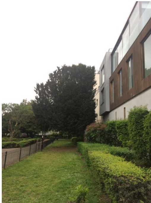
Photograph 2 – Existing clearance between T1 and building
