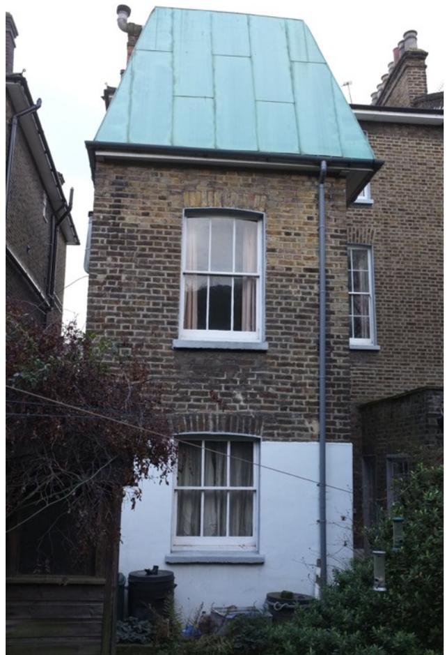
Rear view, showing the existing copper clad mansard extension above the original two storey outrigger.
