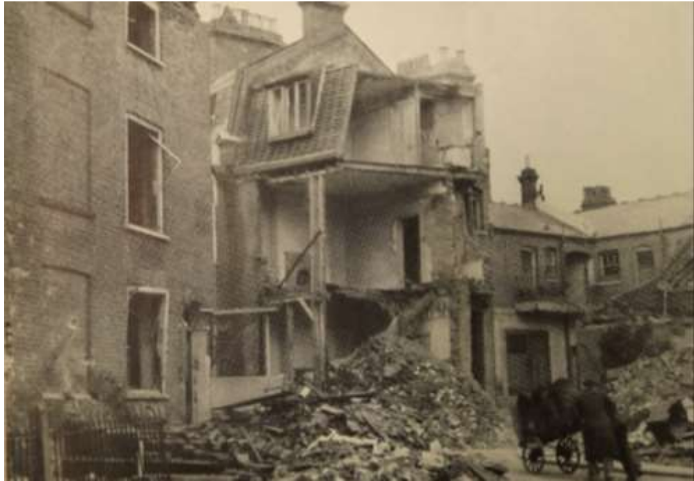
Figure 8: Undated photo showing extent of WWII damage (16 New End Square on extreme left of image)
