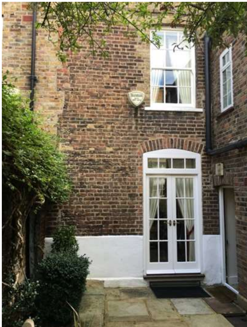
Figure 12: Original part of rear elevation
