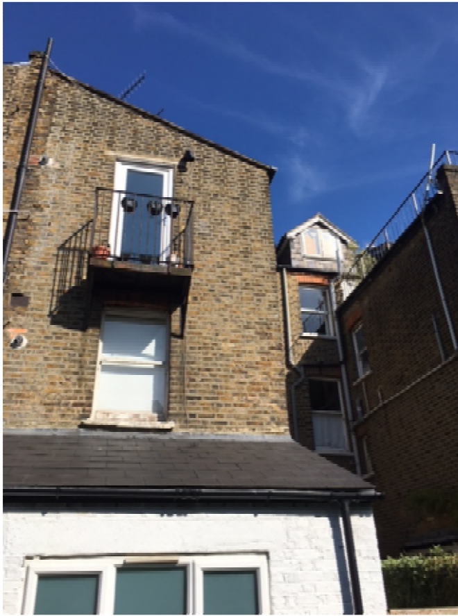
4. Existing dormer at No.66
