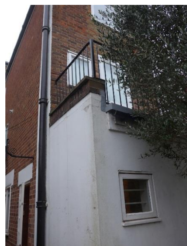
existing rear extension
