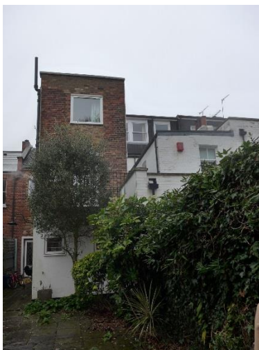
Photographs of the existing rear elevation
