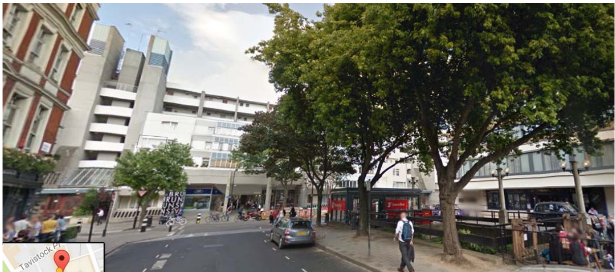
View of the standalone structure with the Marquis Cornwallis PH on the left hand side and the listed Brunswick Centre at the back – both are within the Bloomsbury Conservation Area, and the hotel on the right hand side.
