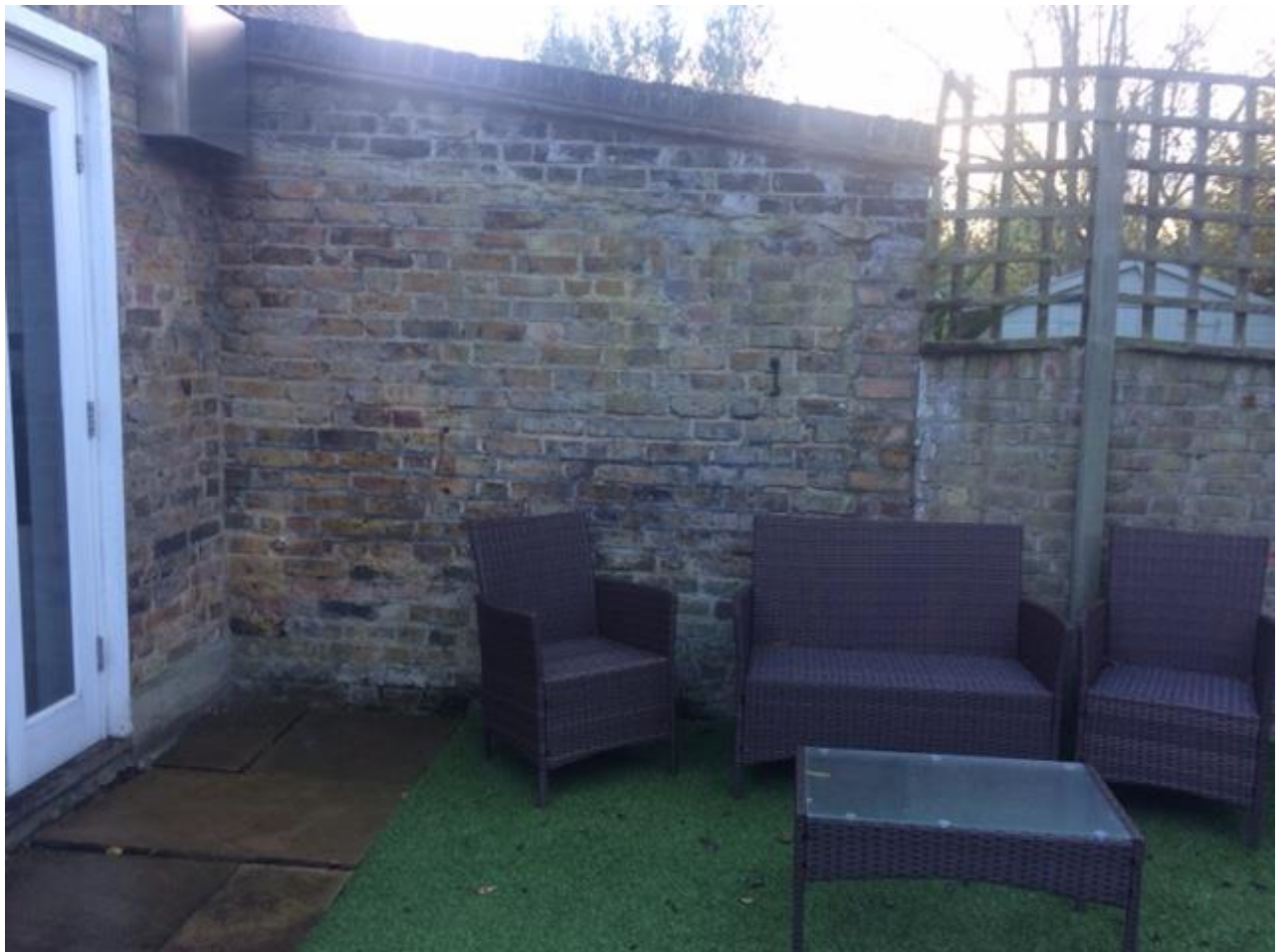
4. View towards the adjacent property at no 57 Solent Road
