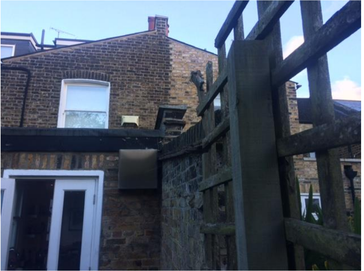
5. View towards the adjacent property at no 57 Solent Road
