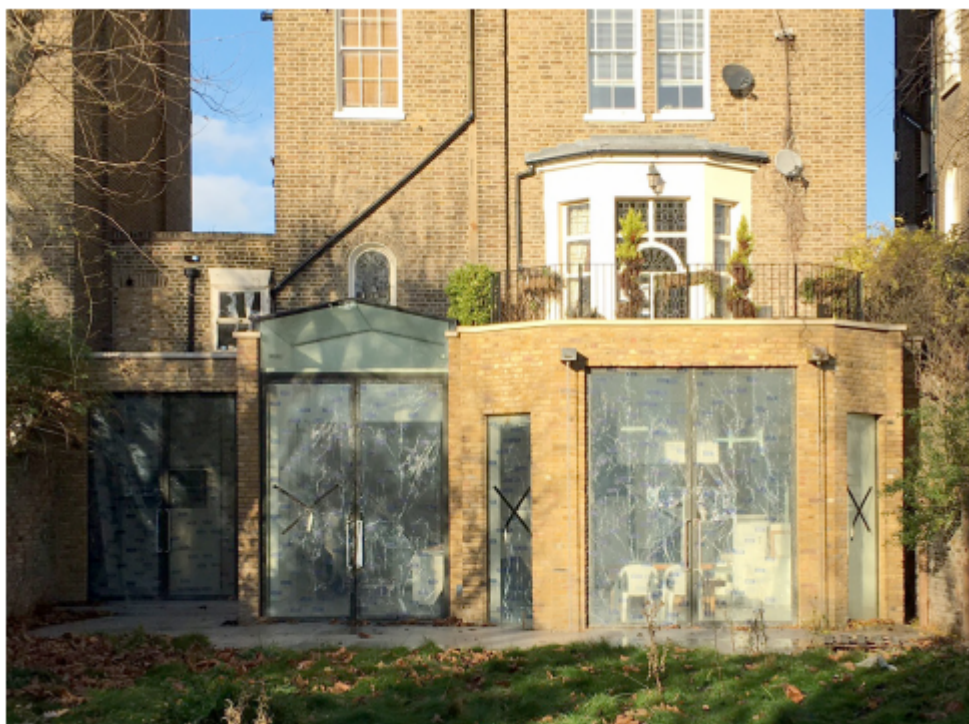
Figure 4 – Rear elevation of adjacent property at 137 King Henry's Road
