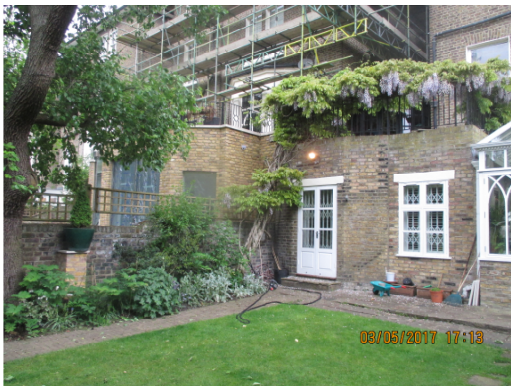
Figure 2 – Showing site in context with adjacent property at 137 King Henry's Road
