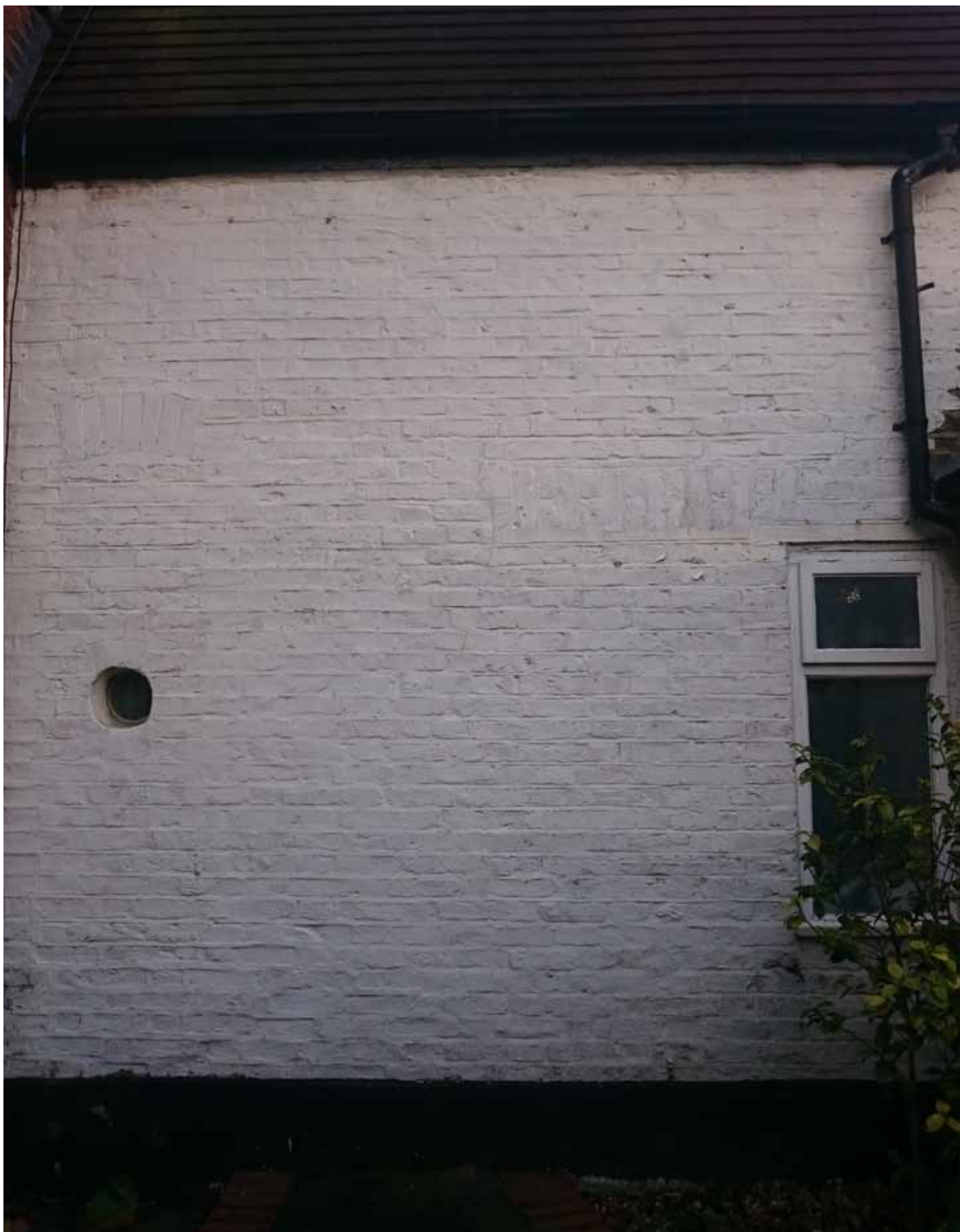
above: East (side) elevation of flat 1. The porthole is located where the new link door is proposed. Traces can be seen of a larger original opening in that location, as well as a 2nd large opening more centrally.
