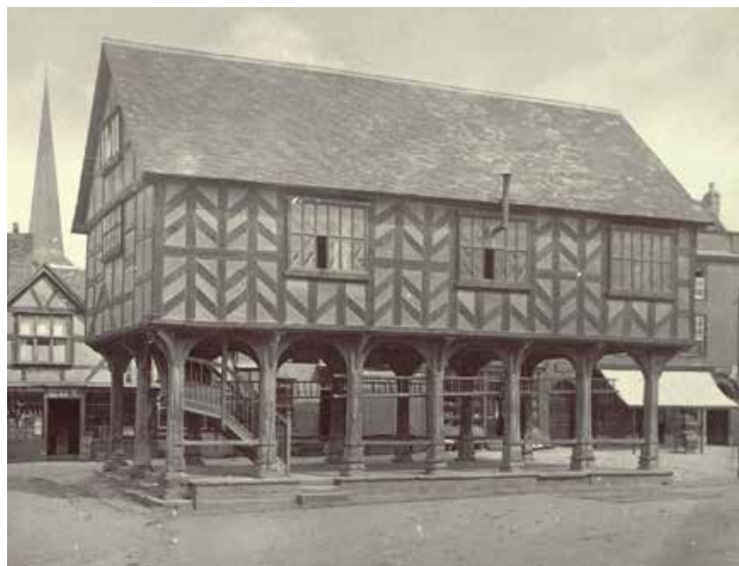
Figure 8: The Ledbury Building
