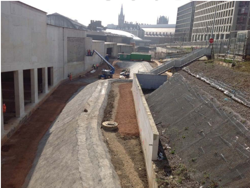
Figure 5 Current view of Sub-Area 4 looking south
