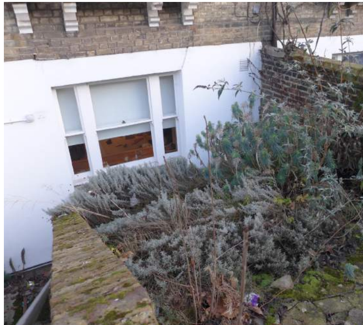
View looking down into the front light-well.
