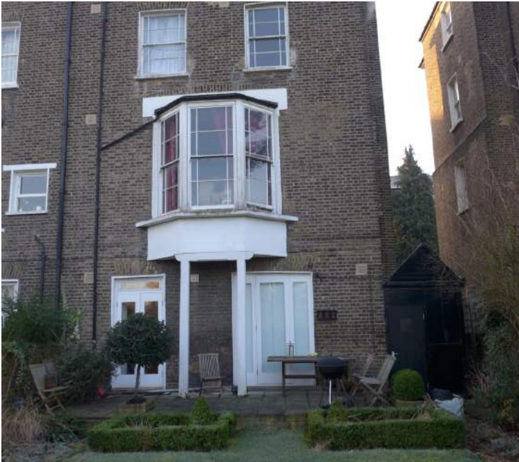
Rear Elevation with level access on to the garden.
