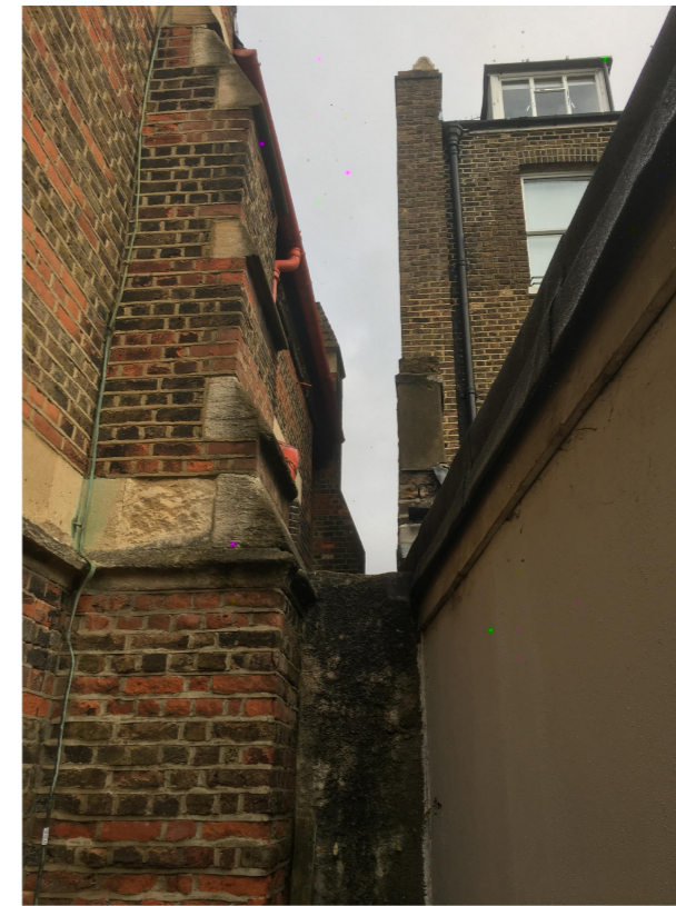
BOUNDARY CONDITION BETWEEN #45 AND CHURCH - AT REAR
