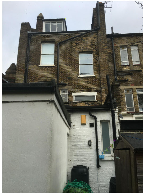
REAR ELEVATION OF #45
