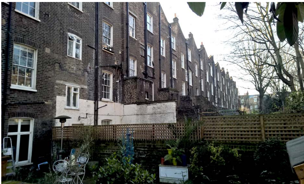
Figure 12/ Original 2 storey stepped rear extensions along Greenland Road
