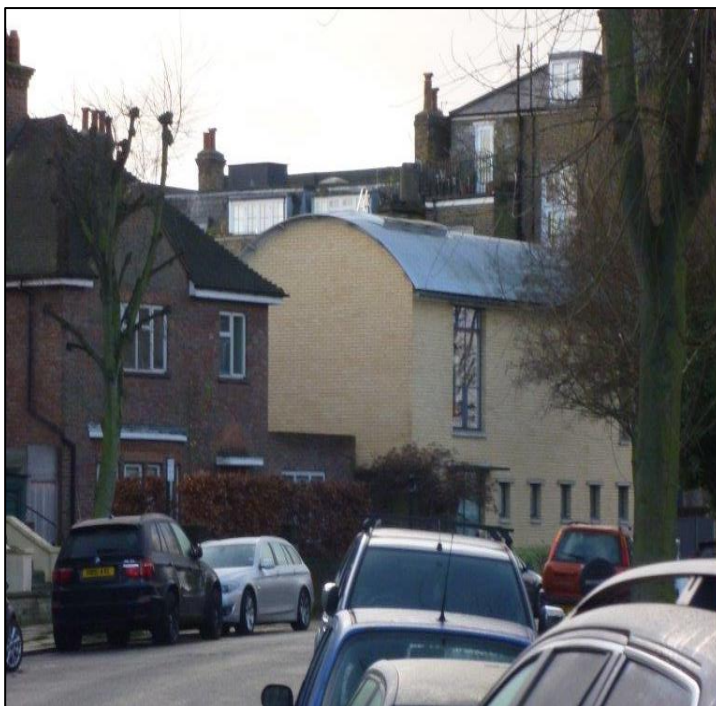
Figure 6. View of the mansard roof of Grove End House from Dartmouth Park Road.
