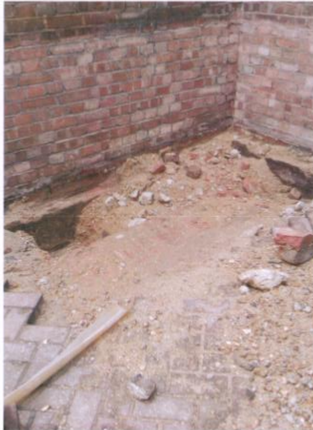
View of the findings encountered in Trial Pit No 5, looking northwest
