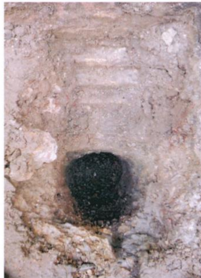
View of the footings encountered in Trial Pit No 2, looking south
