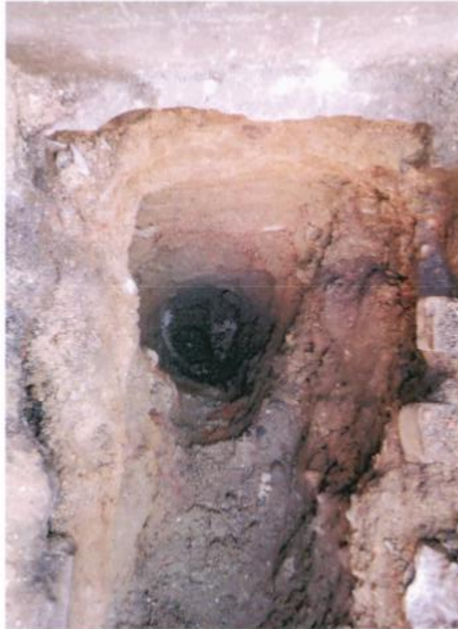
View of the footings encountered in Trial Pit No 3, looking south
