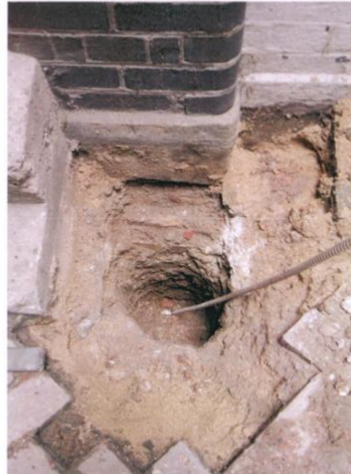
View of footings encountered in Trial Pit No 1, looking east
