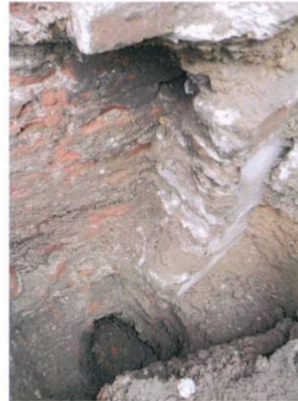
View of the footings encountered in Trial Pit No 4, looking northeast
