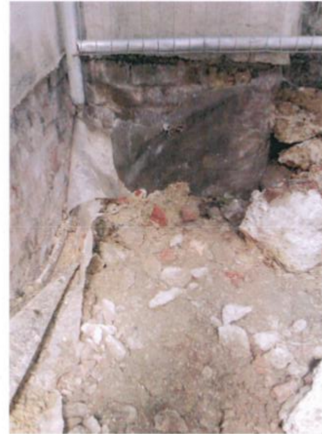
View of the findings encountered in Trial Pit No 6, looking north
