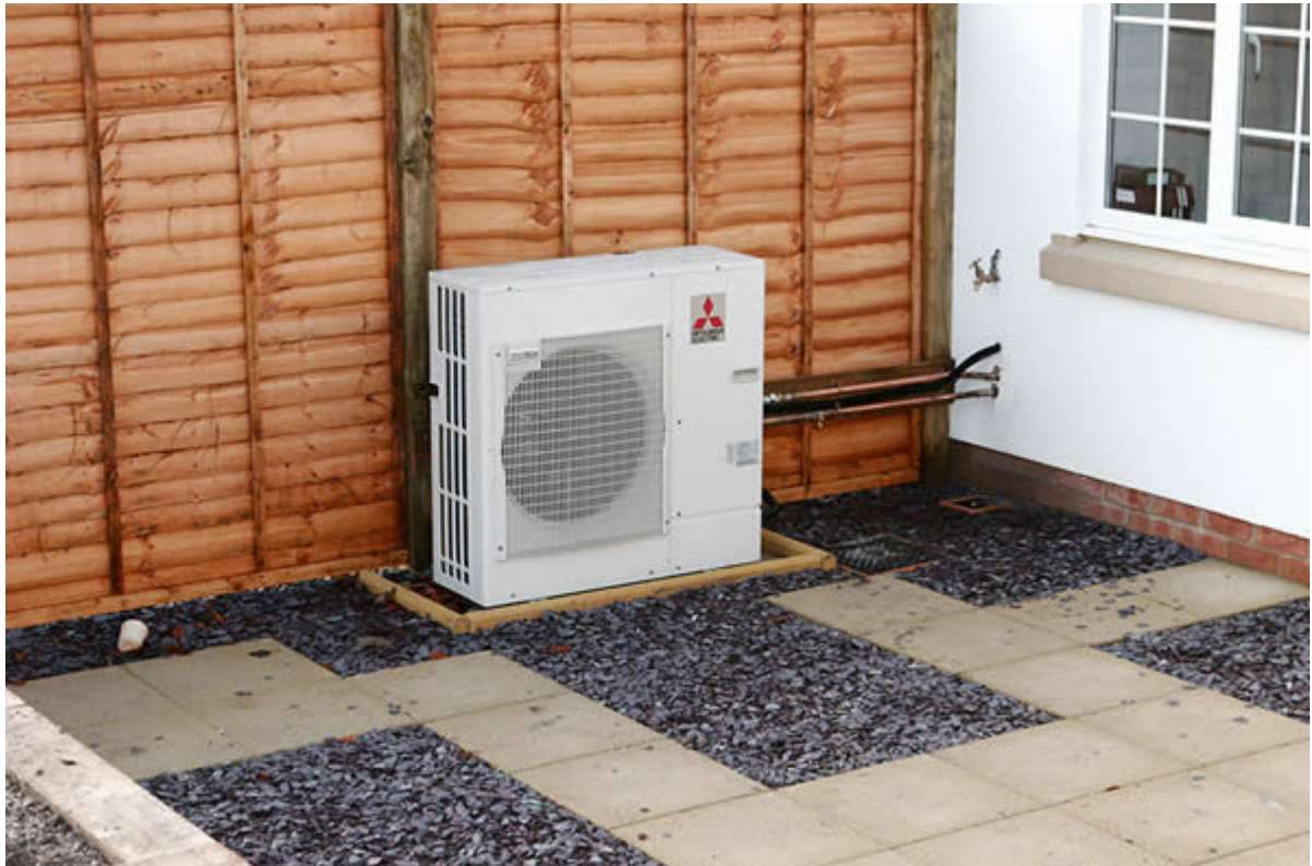
Figure 16 – Typical Air Source Heat Pump External Condenser
