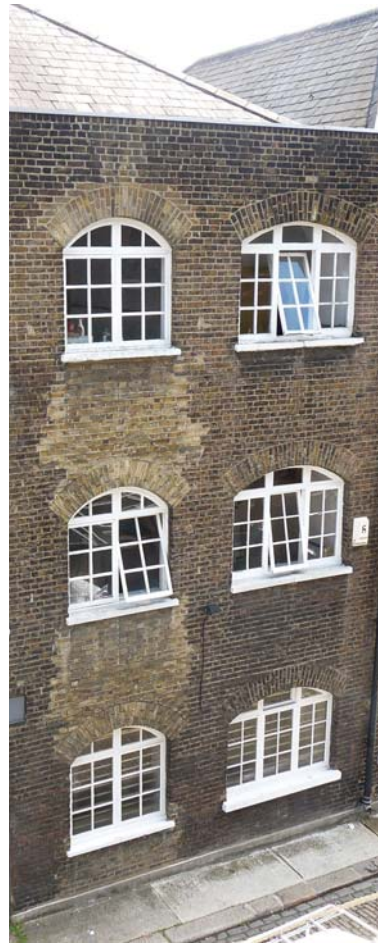
Evidence of historical hoistway on existing building's facade.
