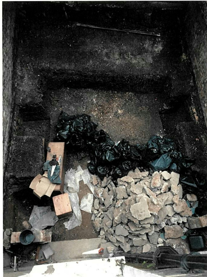
Fig 1 - foundations in rear garden, photo from 30 April 2017
