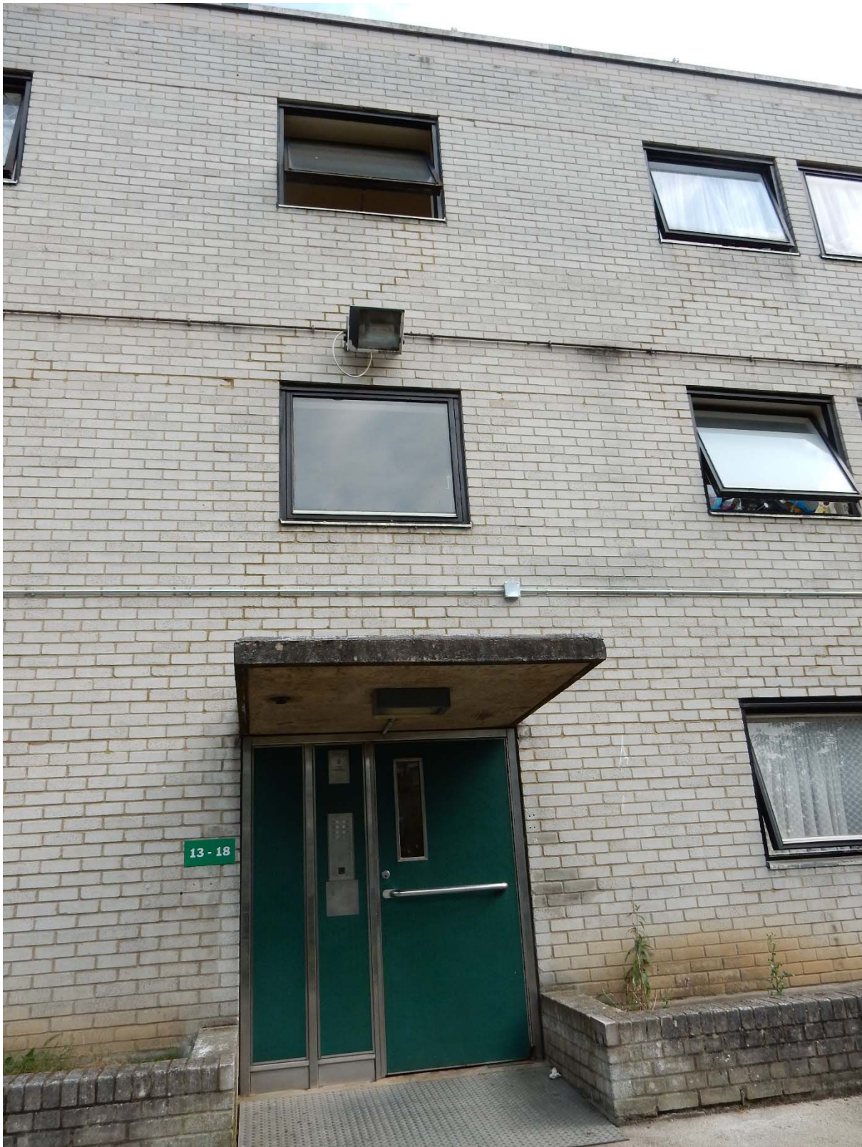
LUDHAM - VIEW OF TYPICAL FRONT ENTRANCE, PRIOR TO WORKS
