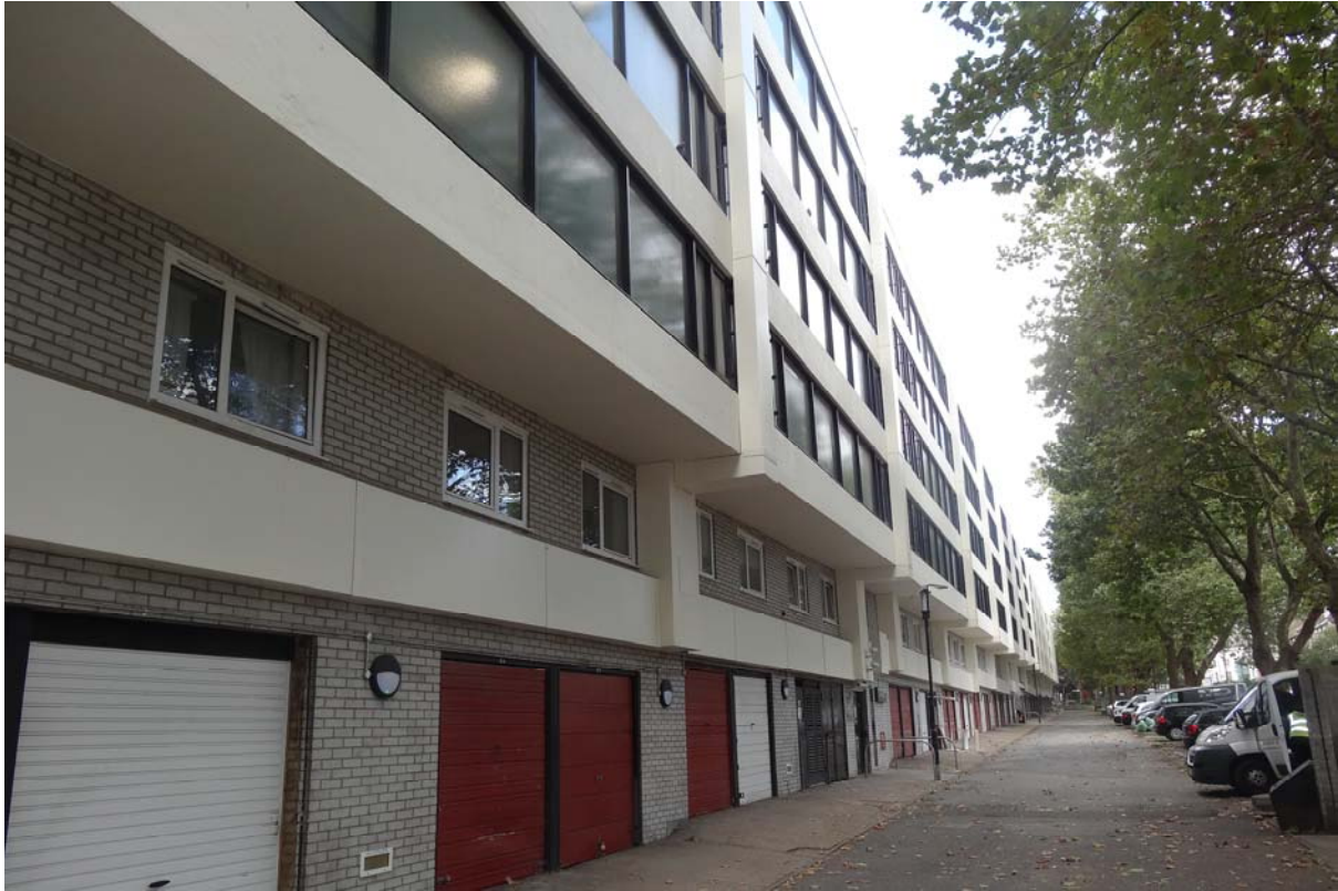
WAXHAM – REAR ELEVATION (FACING WEST) WITH CLADDING COMPLETED
