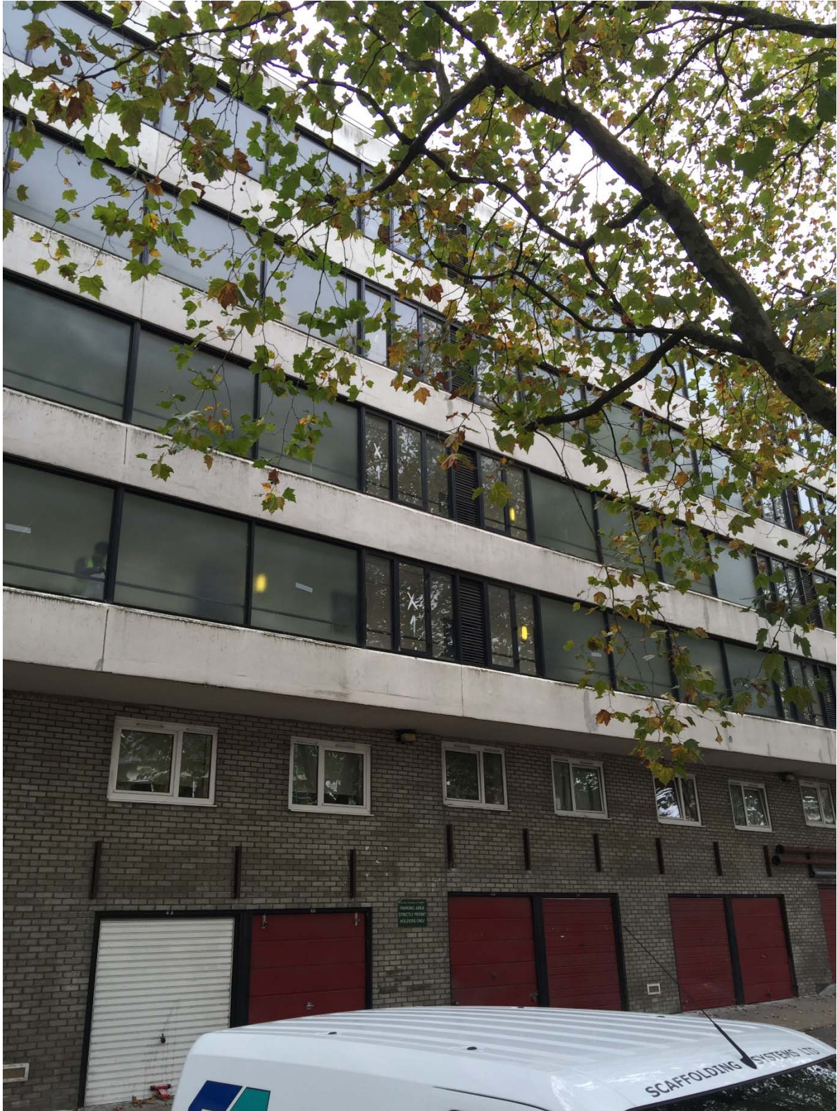
WAXHAM - VIEW OF PARTIAL REAR ELEVATION, PRIOR TO WORKS
