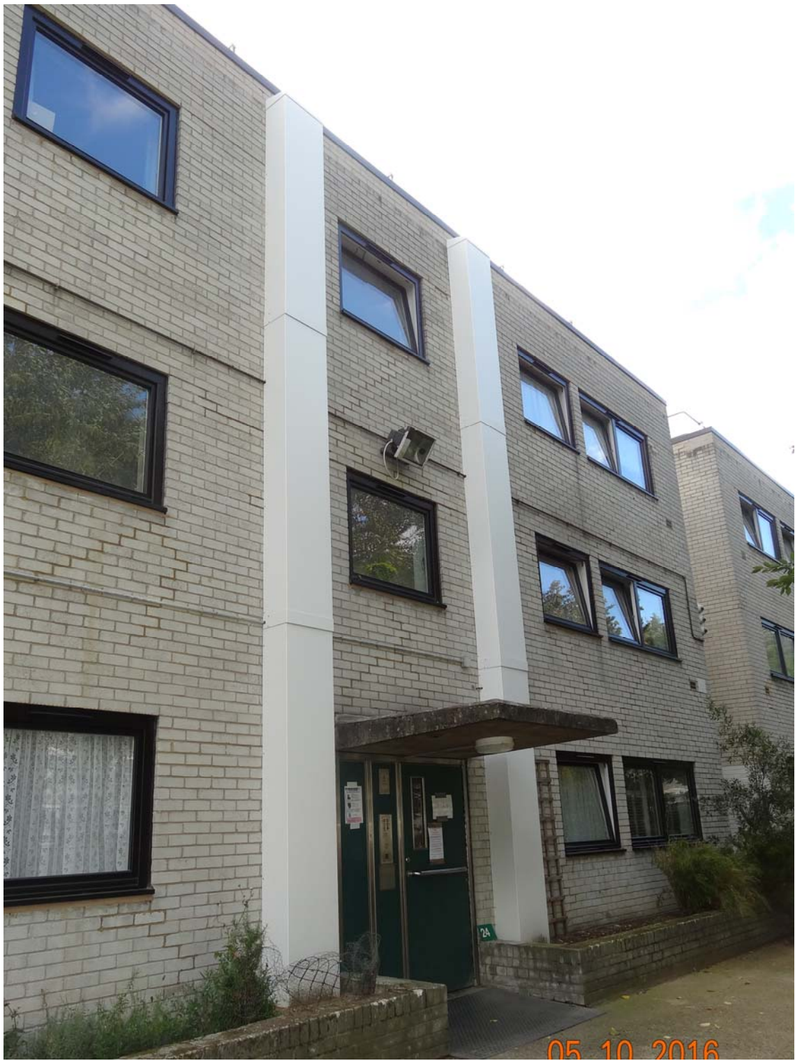
LUDHAM - WITH CLADDING COMPLETED
