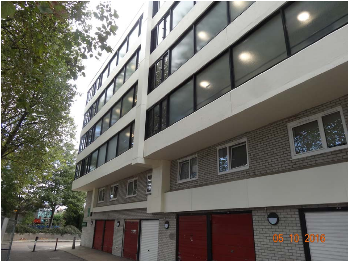
WAXHAM – REAR ELEVATION (FACING EAST) WITH CLADDING COMPLETED
