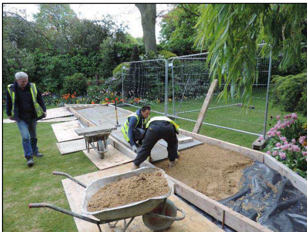
Photo 1: Concrete paving slabs being laid.
