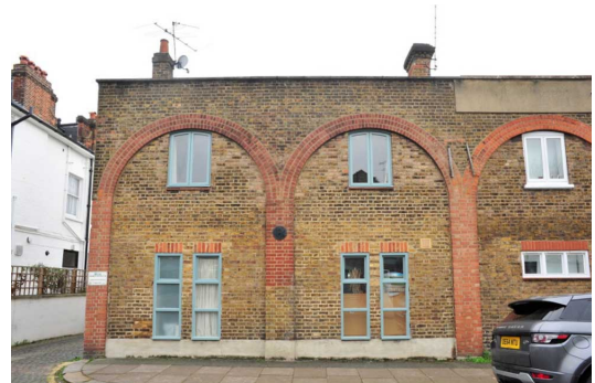
Photo of existing rear elevation facing Lambolle Place
