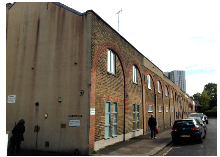
Photo of existing rear elevation facing Lambolle Place
