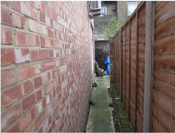
fig. 6 Garden alley between existing extension and 88 Parkway
