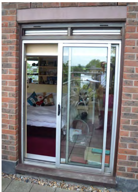
Existing timber surround and aluminium frame double glazed doors
