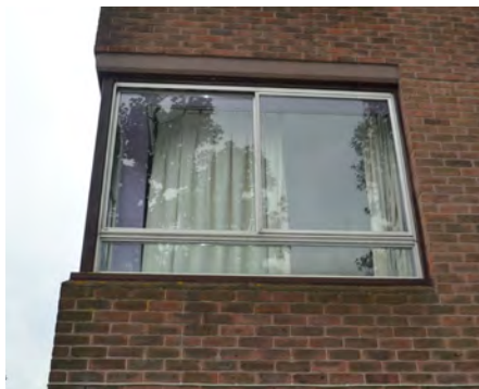
Existing timber surround and aluminium frame double glazed windows
