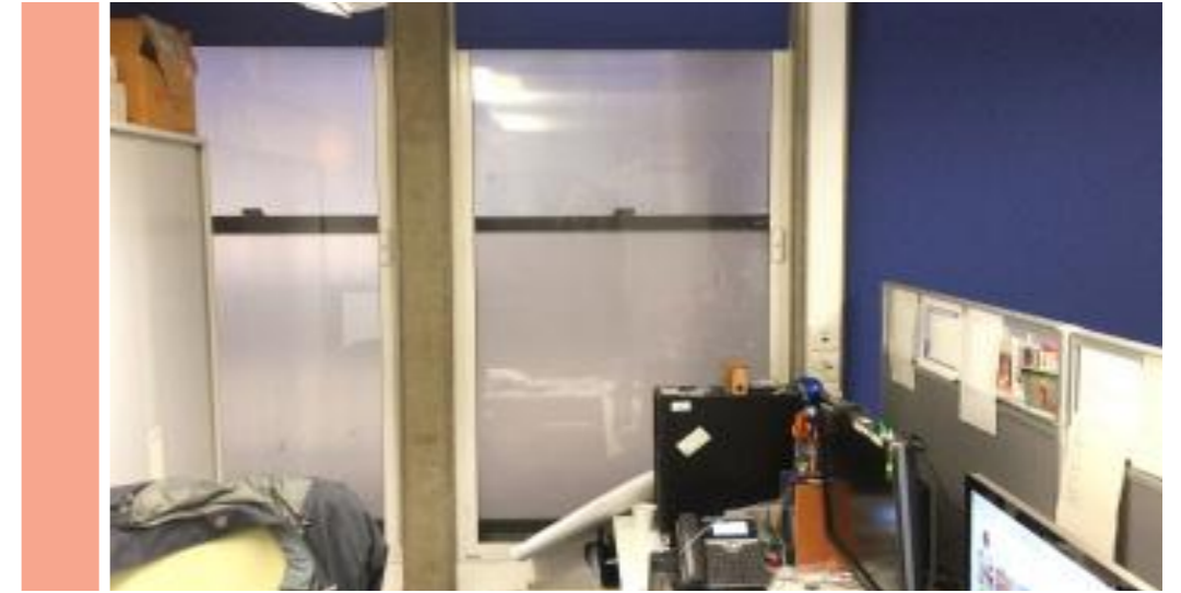
Photo showing existing secondary glazing (Type 2) to be replaced with new
