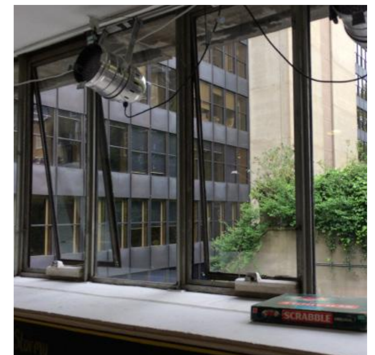
Windows Level 3 wing window to be replaced
