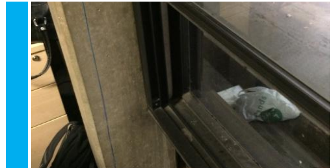
Photo showing existing secondary glazing (Type 1) to be replaced with new
