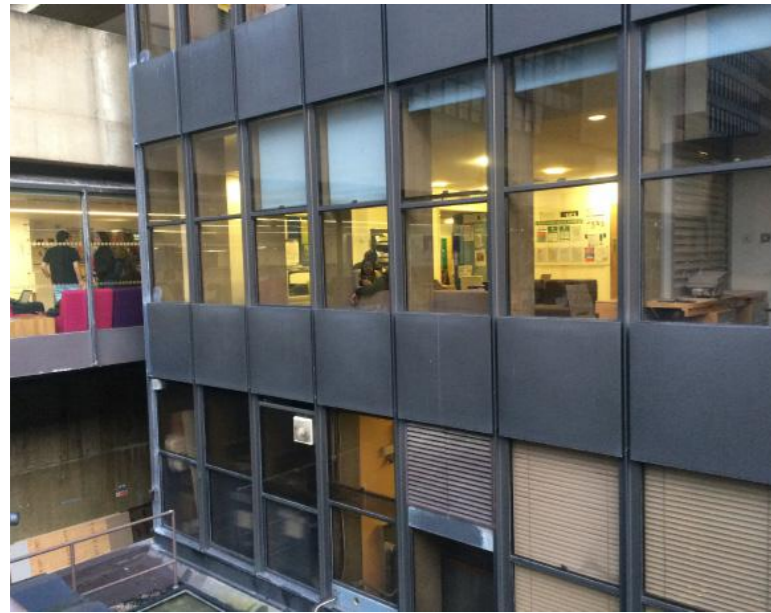
The photo above is taken from the external square, and illustrates that the proposed lift will essentially not be visible due to its distance (~3m) away from the windows. The lift shaft will appear similar to an internal room, and it will also be obscured by the concrete mullions.
