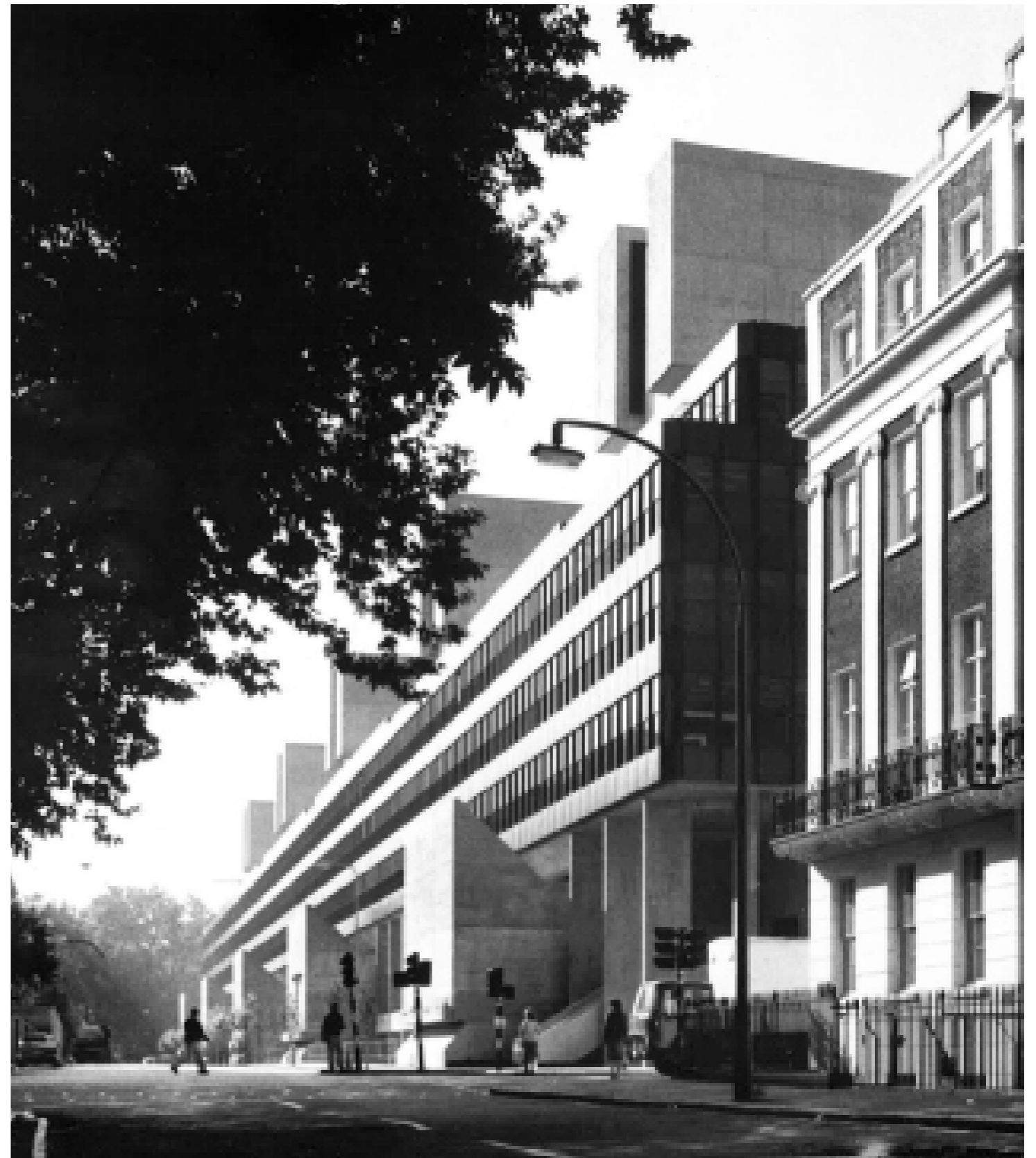
Right: Image from 1977 showing intent of cladding to reflect vertical proportion of surrounding Georgian terraces
