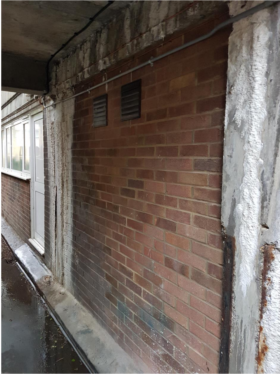
The exit for the extractor fan – the first black grate in the picture.
