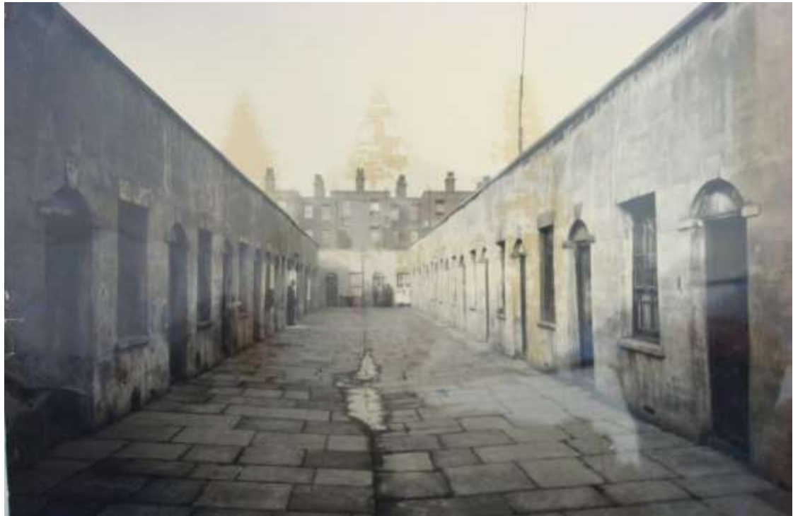
Figure 7: Equity Buildings, Looking North, 1928
