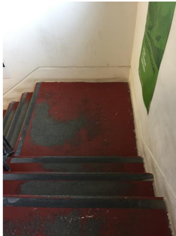
Plate 9: Principal staircase treads change colour as one moves up the building
