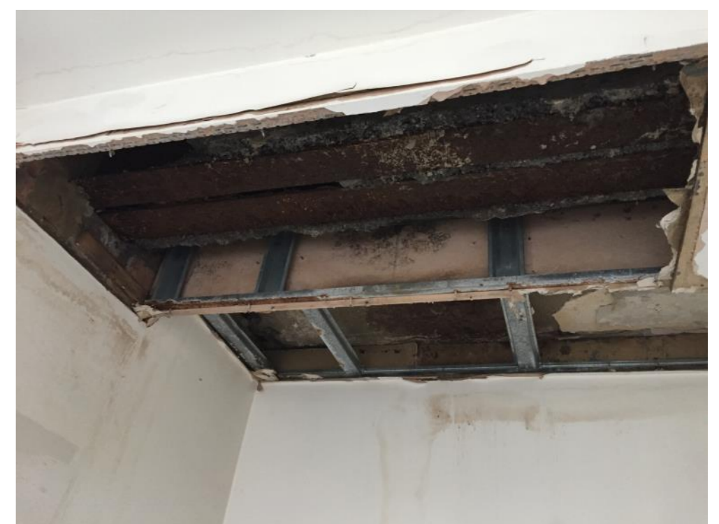
Plate 11: Steel Frame structure above plaster board ceilings at 6th floor
