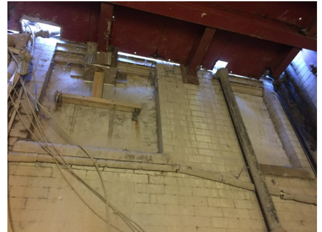
Plate 7: Remnant of rear elevation within lightwell at Lower ground floor level
