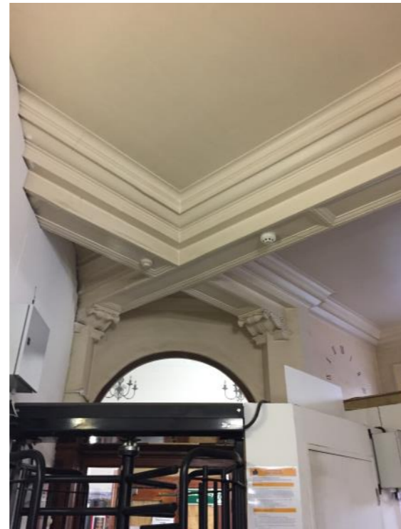
Plate 5: Ground Floor ceiling with replica down stand cornices
